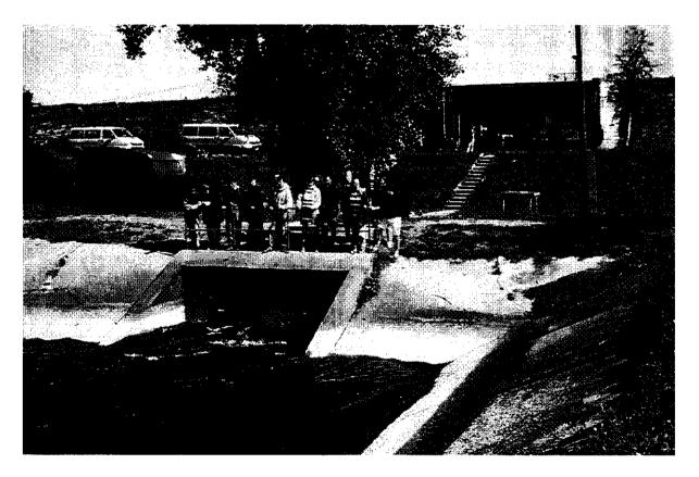
Figure 7 The intake structure. Behind the dyke is the reservoir.
