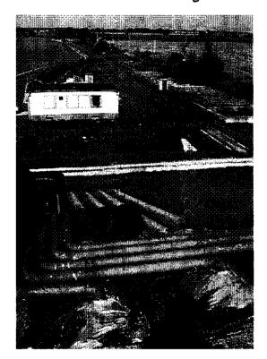
Figure 12 Inlet of water from the canal by means of syphons
