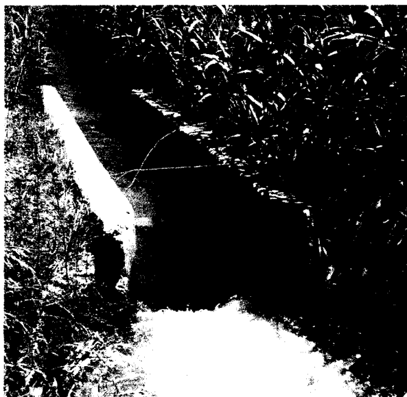
Figure 8.4 The actual volume of water flowing through an irrigation canal can be measured accurately with a long-throated flume (Bos 1976; Clemmens et al. 1994)
