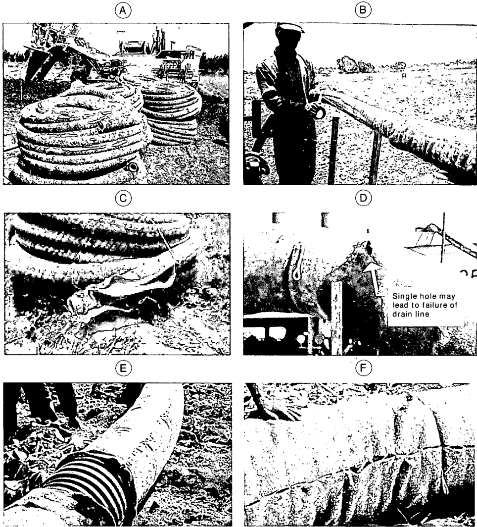
Figure 21 Improper wrapping, stitching and handling of envelopes.
