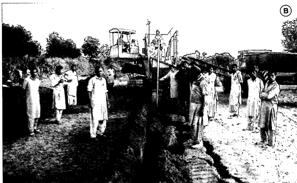
Figure 25 Trench backfill in practice.
