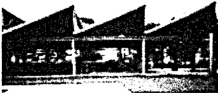
Photo 1: High-tech farm barn roof
