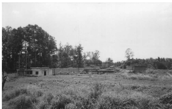
The existing wastewater treatment system of Bien Hoa Sugar Company
