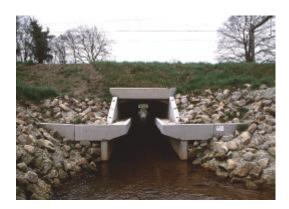
Figure 8. Ledges on both walls of a culvert enables newts to pass infrastructure (Photograph: Edgar van der Grift)
