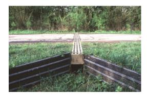
Figure 7. Small fauna underpasses proved to be effective means to help amphibians cross roads safely (Photograph: Edgar van der Grift)
