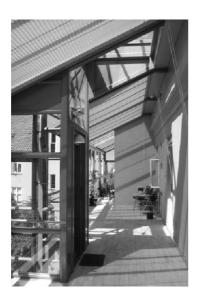
Figure 6. Another urban renewal demonstrations project where broad recreational balconies and an elevator were built outside the facade of an existing building. In this case one elevator gave access to more staircases. (http://www.paalsson.dk/)
