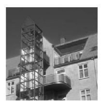
Figure 5. Urban renewal demonstrations project where small balconies and an elevator have been installed. The elevator was installed because new flats were made in the attic. Thereby also the other flats got access by an elevator. (http://www.paalsson.dk/)
