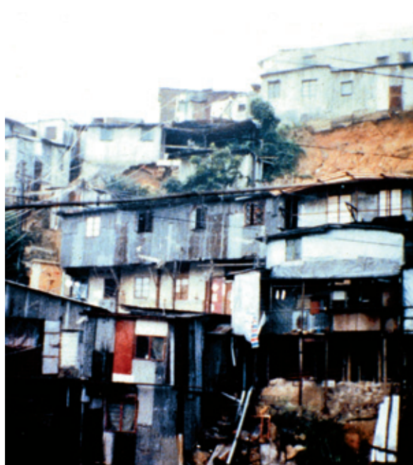
Urban development on steep land in Hong Kong. Aerial view of the same site after a landslide triggered by heavy rains.
