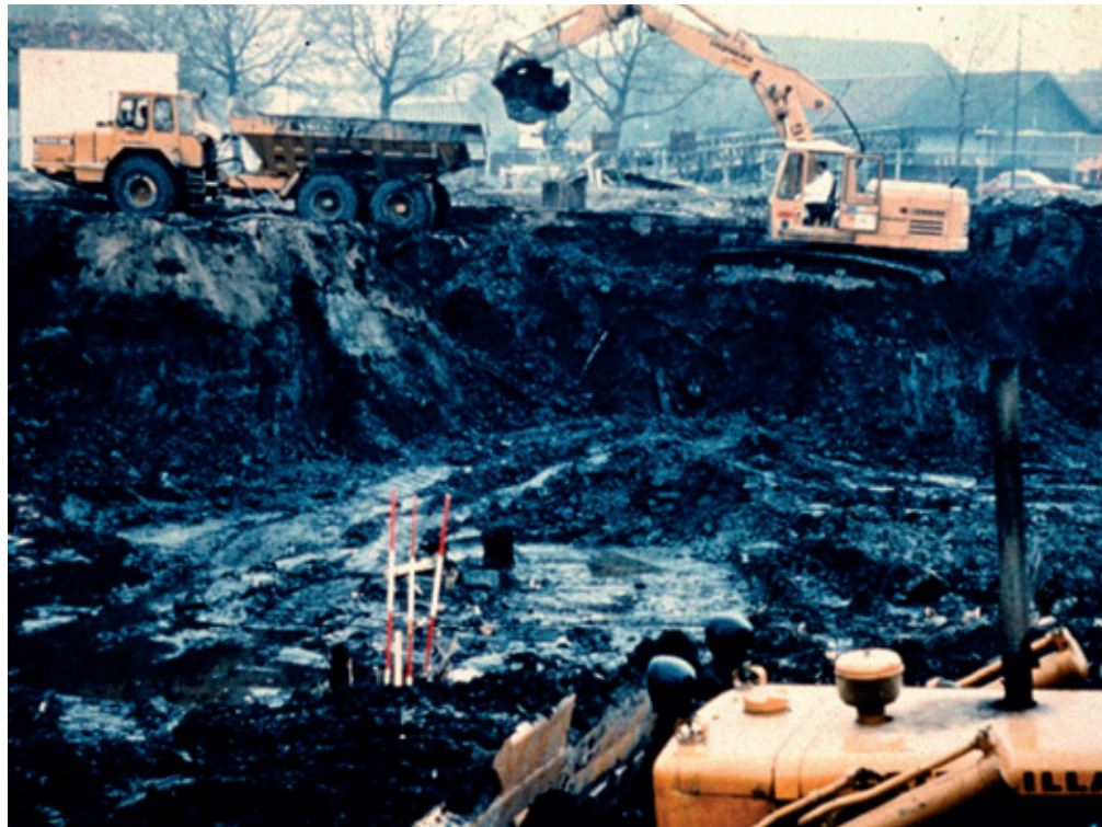
Severely polluted soils in the Netherlands for which excavation is essential
