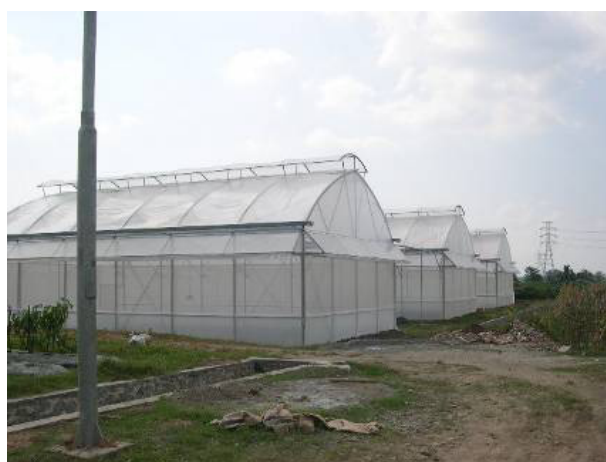
Figure 26. The Greenhouse construction at Purwakarta.
