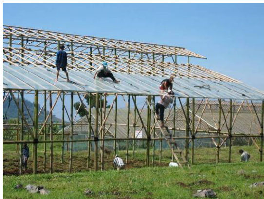
Figure 27. Bamboo plastic house under construction.
