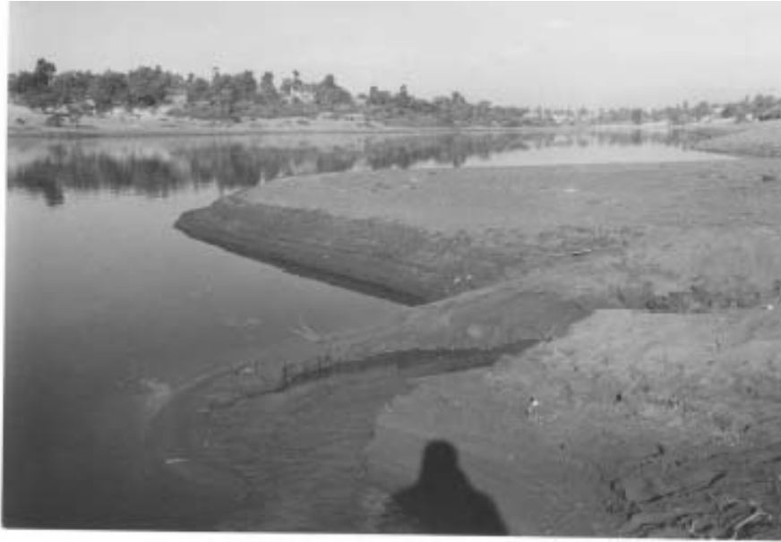
Figure 2.6. Sediment load transported by a stream into the hydropower reservoir in Fincha'a watershed, western Ethiopia. (Photo: February 2003)
