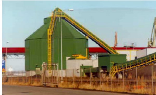
Fig.23. The round-bottom intermediate storage ( 1500\text{ m}^3 ) of a biofuel power plant, Source [47]
