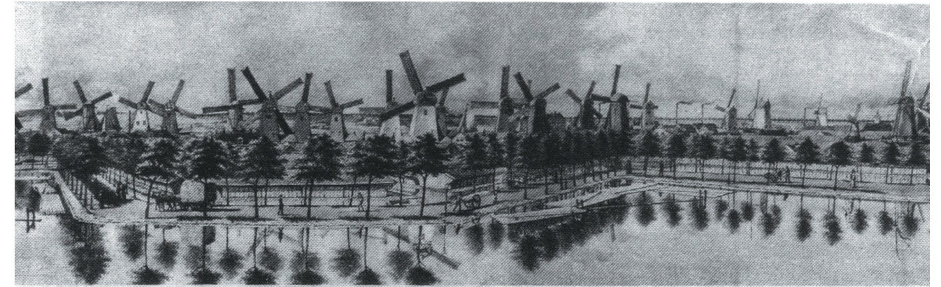
Windmills in Amsterdam; sustainable water management in first half of the 19th century.
