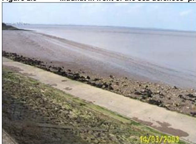
Figure 2.3 Mudflat in front of the sea defences- prior to inundation
