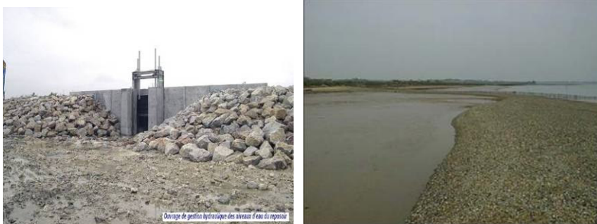
Figure 1.4. Technical measures for habitat creation and restoration. Left: sluices at the Seine estuary after construction (France); Right: artificial foreshore creation at Shotley (UK)
