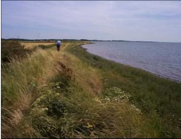
Figure 10.3 West Chidham, prior to scheme construction
