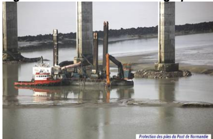
Figure 25.5 Normandie bridge piers protection
