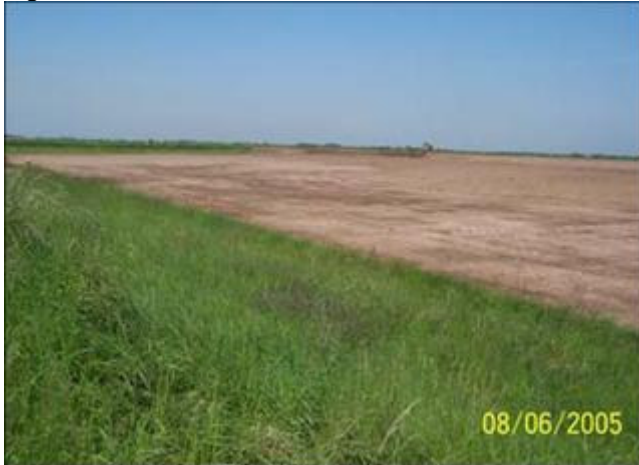
Figure 9.2 The Welwick site under construction
