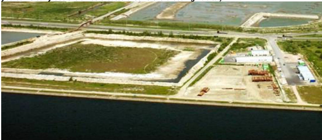
Figure 15.2 Gull breeding habitat at Deurganck dock after implementation of the scheme (on the left you can clearly see the dikes created around the breeding habitat)
