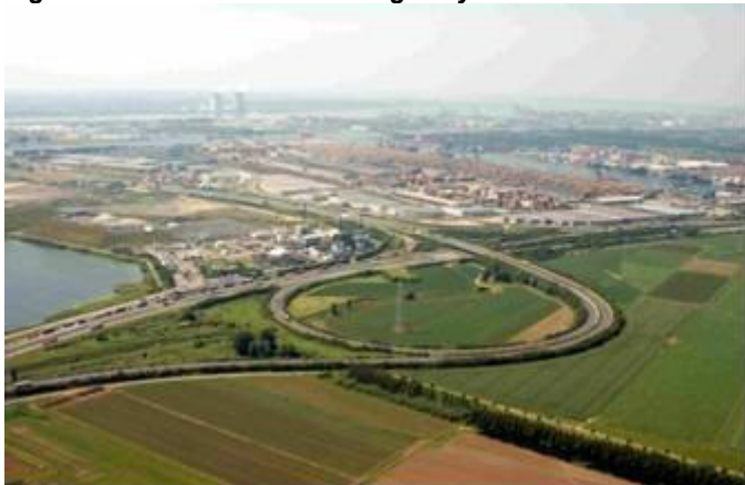
Figure 16.1 The A12/R2 highway intersection before implementation of the scheme.
