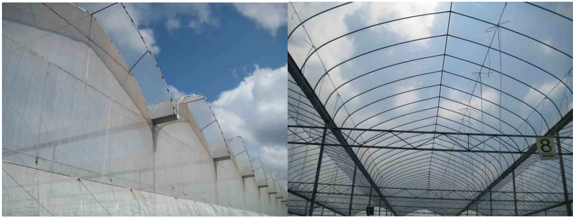
Figure 5. Terengganu greenhouses with gothic roof system and without top opening.
