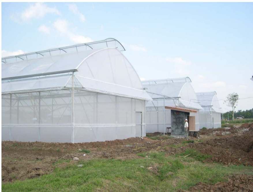
Figure 7. Greenhouses with a new foil type (high light transmission, transformation of direct in diffuse radiation, and reflection of heat radiation) and chimney ventilation constructed at East West at PT East West Seed Indonesia (EWINDO) in Purwakarta, Indonesia.
