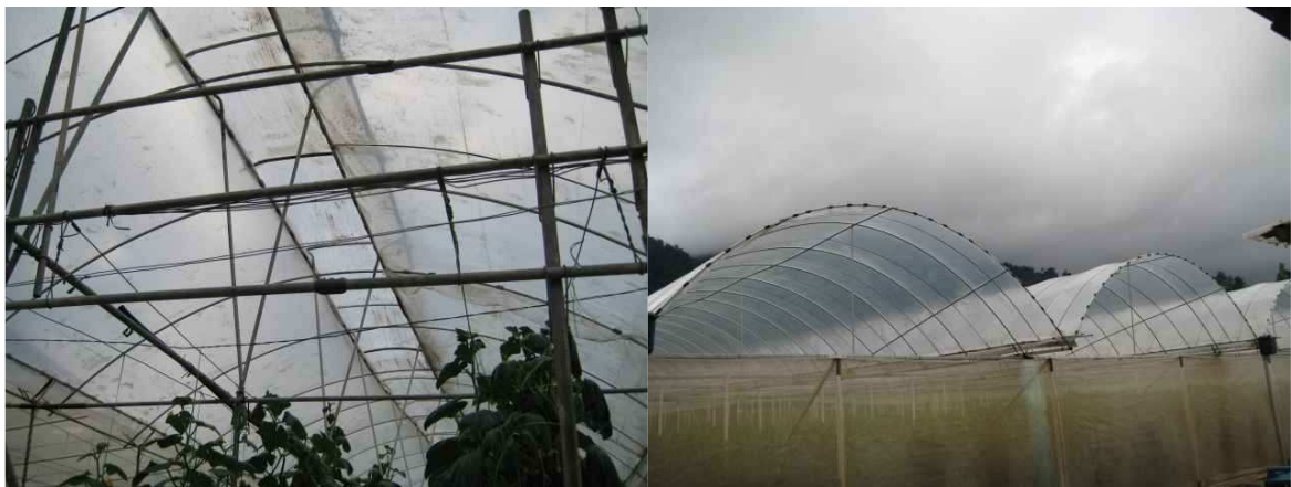
Figure 6. A traditional greenhouse design with a top opening (left), and a traditional greenhouse design without a top opening, as found in most greenhouses in the highlands (right).
