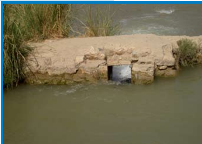
Photo 12. Aliabad Canal, Kunduz Province
