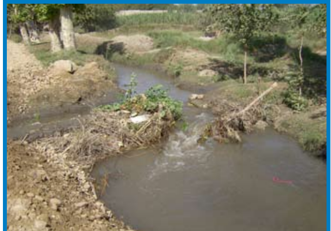
Photo 6. Kama Canal, Nangarhar Province
