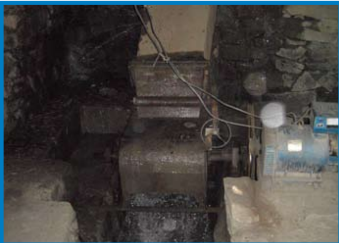
Photo 20. Pacha Joi Canal, Laghman Province
