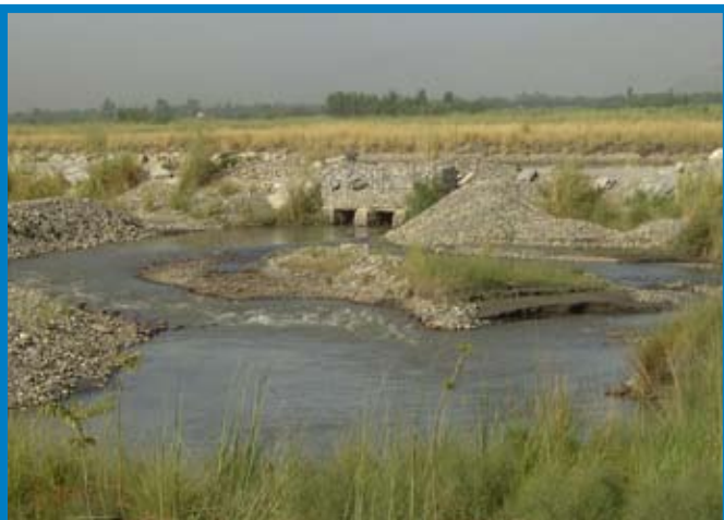
Photo 27. Kama Canal, Nangarhar Province
