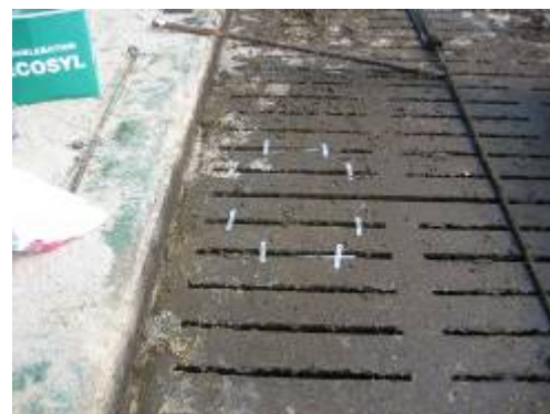
Figure 2 Separating a part of the slurry pit
