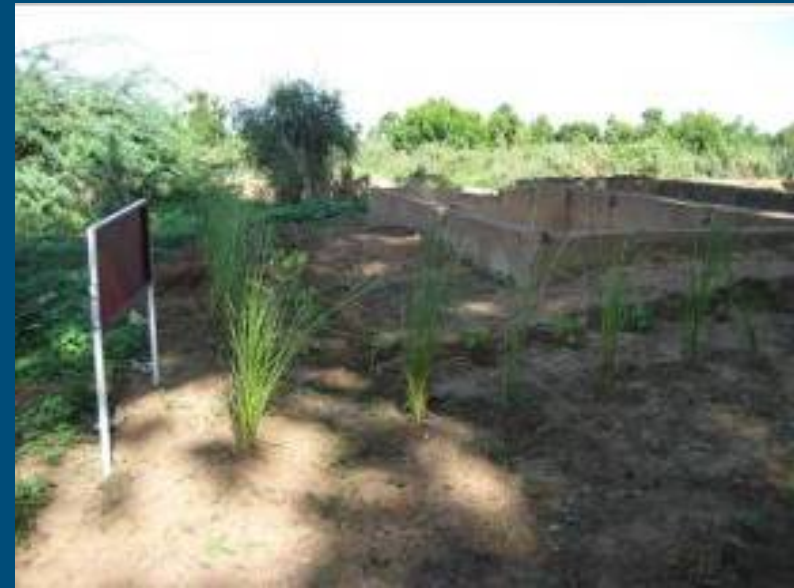
Fence vegetation around depot
