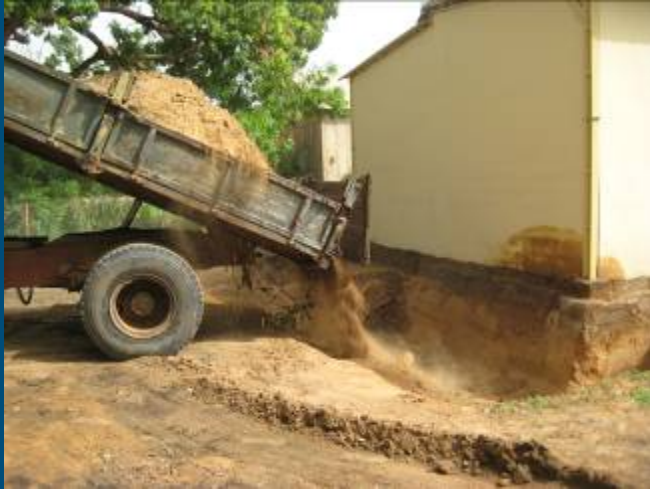
Refilling with active soil
