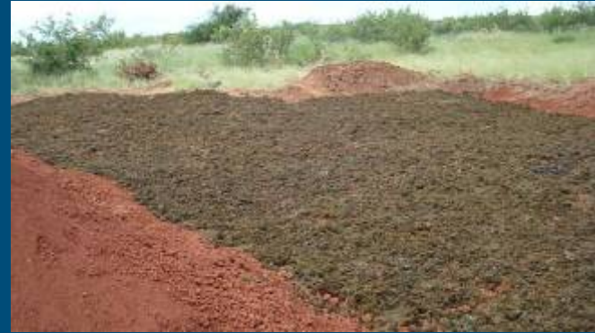
Preparation of landfarm
