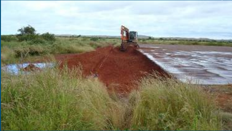
Excavation of source
