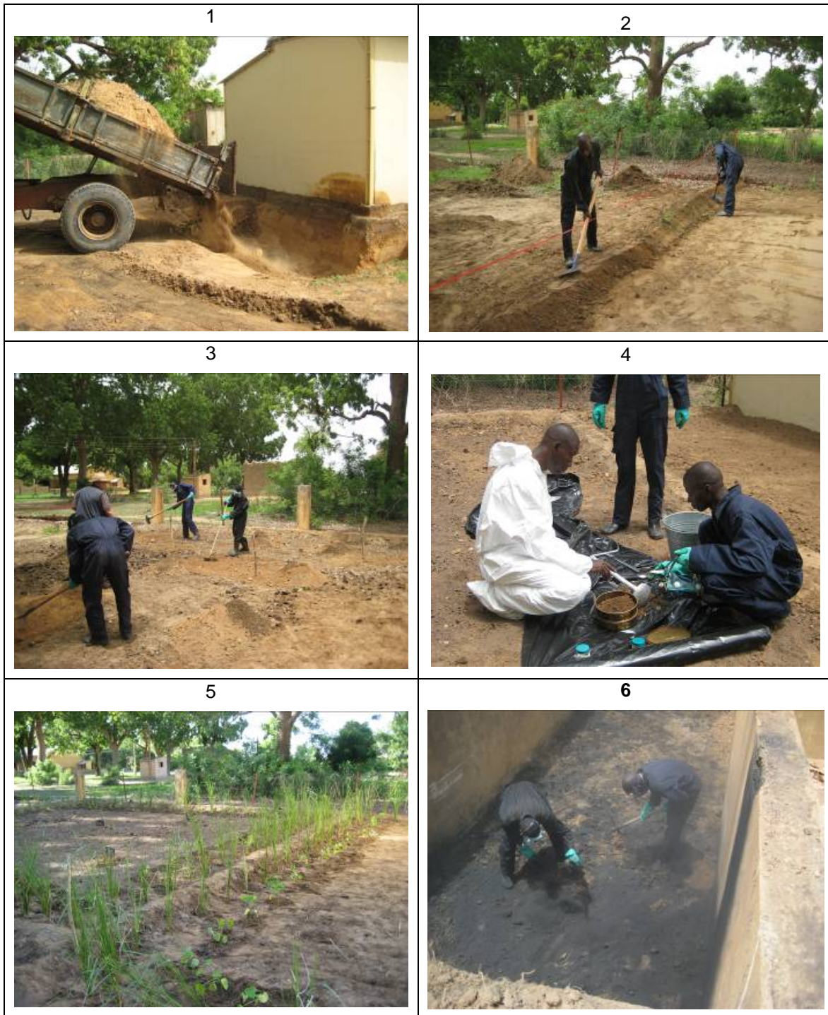
FIGURE 3. Implementation of risk reduction in Molodo. (1) Filling of the excavated center with biological active soil. (2) Making elevations around the landfarm. (3) Mixing the first charge on the landfarm. (4) Sampling on the landfarm. (5) Vegetation on the center area and around the landfarm. (6) Enrichment of soil in the concrete construction with charcoal.
