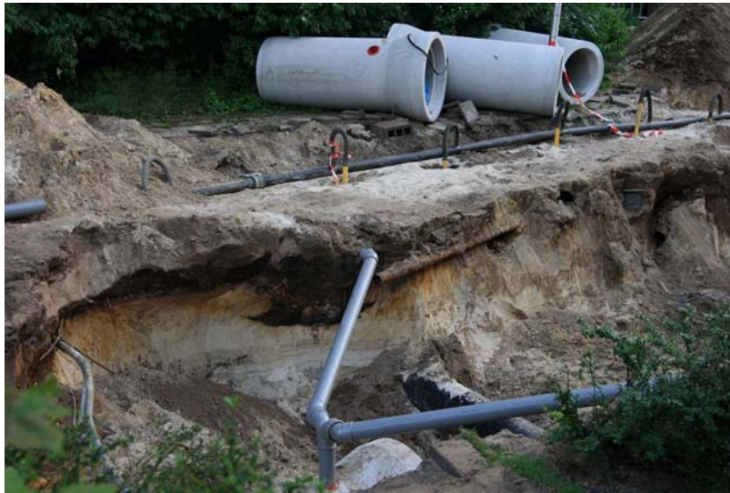
Figure 1.1: A sewer system under construction.
