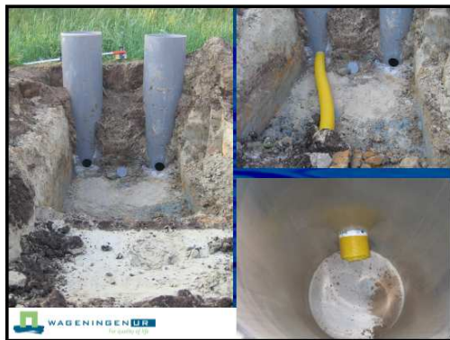
Figure 24 Pipe connectors between (a) field drains and (b) field and collector drains
