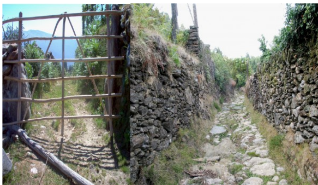
Figure 2. Field path with calçada Portuguesa (Minho, Northern Portugal) as the path between fields to the grazing land with the gate closed (left) and the gate open (right).
