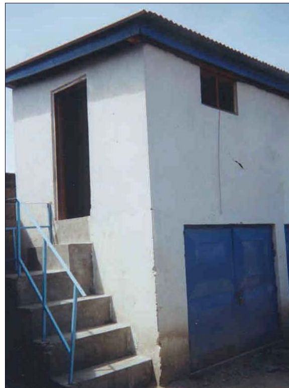
Figure 10 - Anaerobic treatment of black waste(water) in Tanzania, family.
