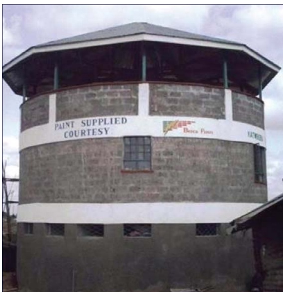
Figure 11 - The SPARC-style sanitation block in Gatwera village in Kibera, Nairobi.
