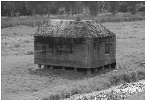
Fig 2.7. An example of the subsidence of a peat soil in the western peat area of the Netherlands. The building is a remaining from the second world war.
