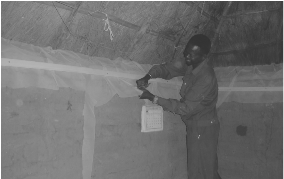
Figure 2.4. Closing off the eaves of a traditional rural house can prevent mosquito entry
