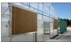
Evaporative cooling with polycarbonate covering
