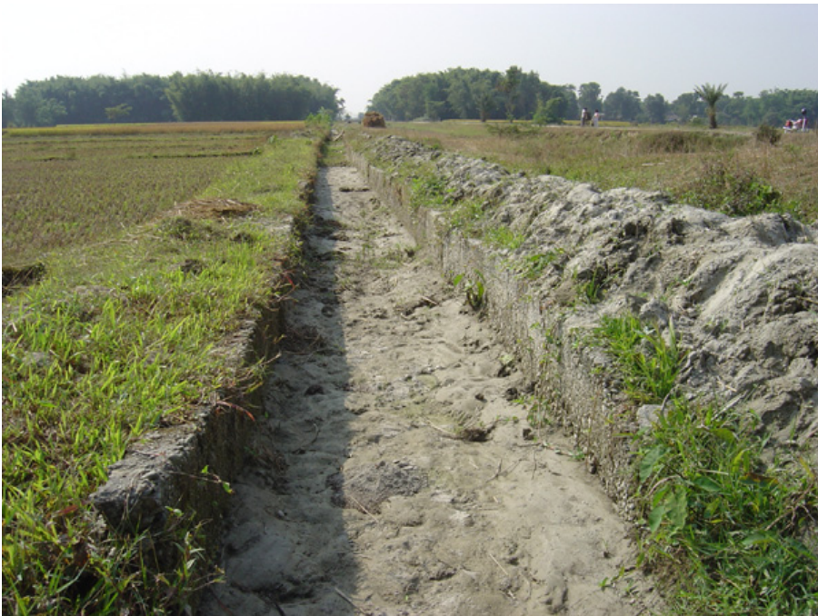
Figure 4.16 Rectangular lined canal with bed deposition.
