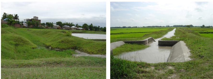
Figure 8.20 Heavily deposited sub-secondary canals.
