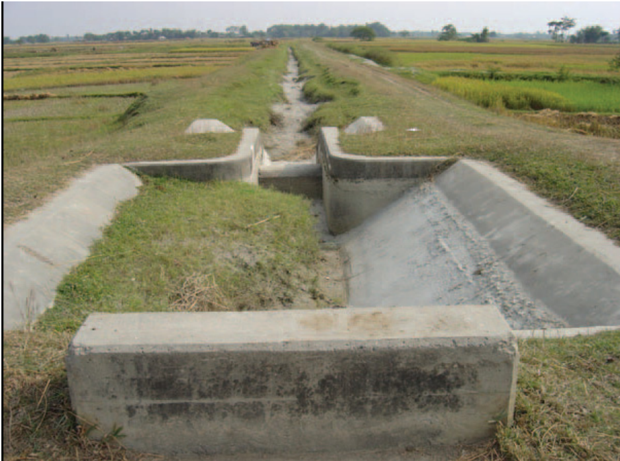
Figure 6.8 Sediment deposition upstream of flow measuring structure. A flume might have been a better measuring structure than a broad crested weir, in terms of sediment transport efficiency.
