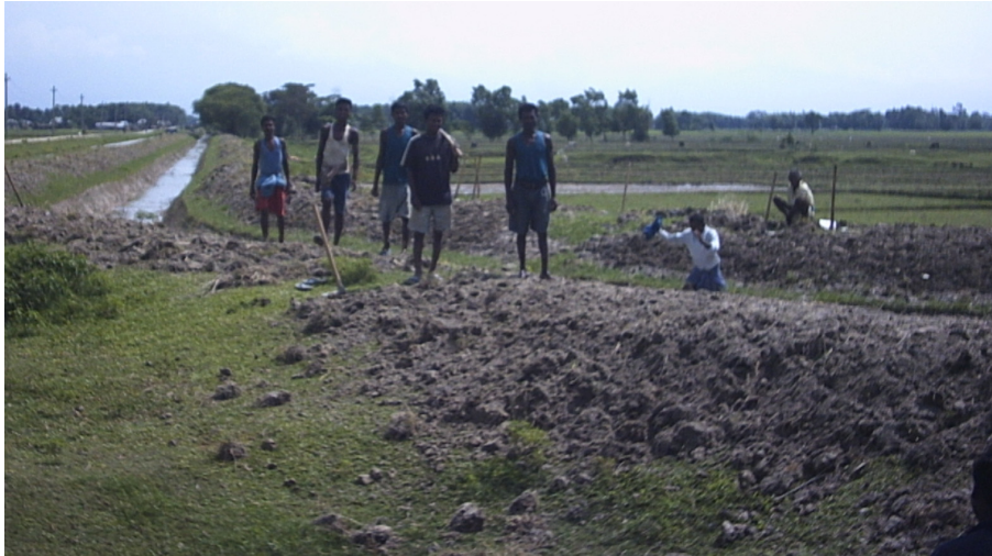
Figure 5.3 Desilting of canal is one of the major maintenance activities.
