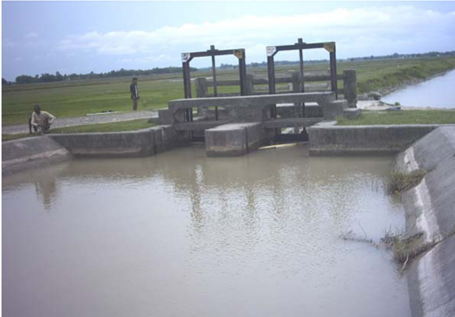
Figure 7.5 Water level regulator in Secondary Canal S9.
