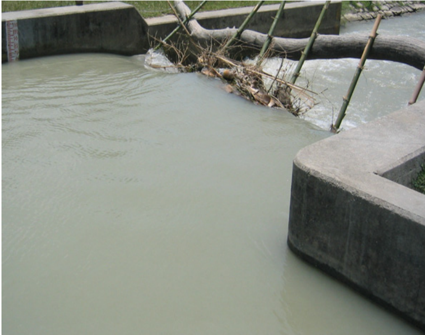
Figure 6.10 Obstruction to raise the water level.
