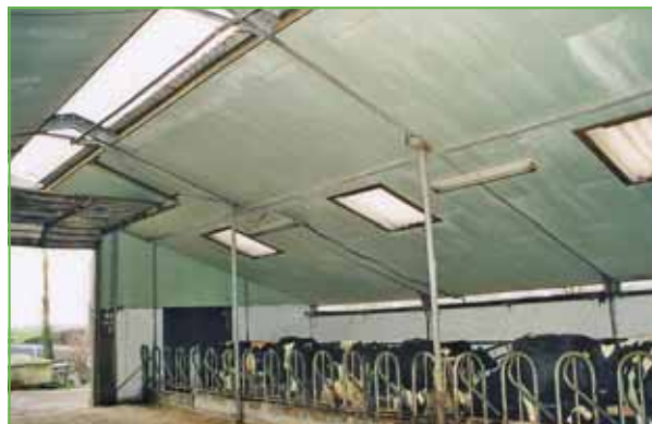
Picture 5. Isolated roofs take care for good indoor climate
