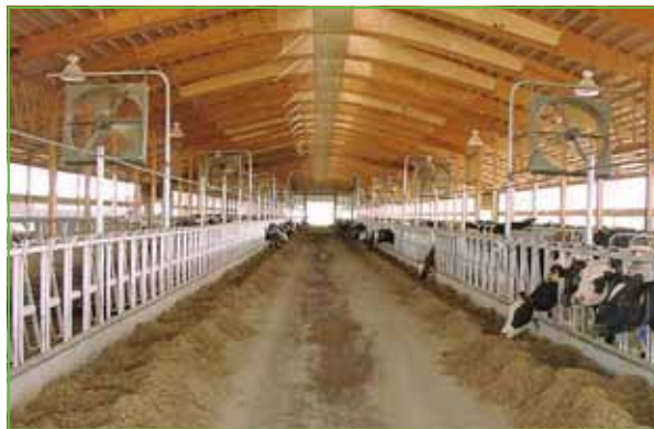
Picture 2. Ventilators for reducing heat stress during hot periods
