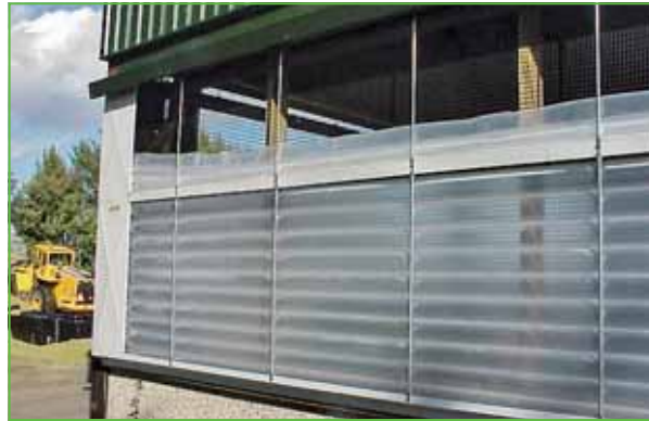
Picture 3. Open side wall with plastic curtains that can be blown up automatically
