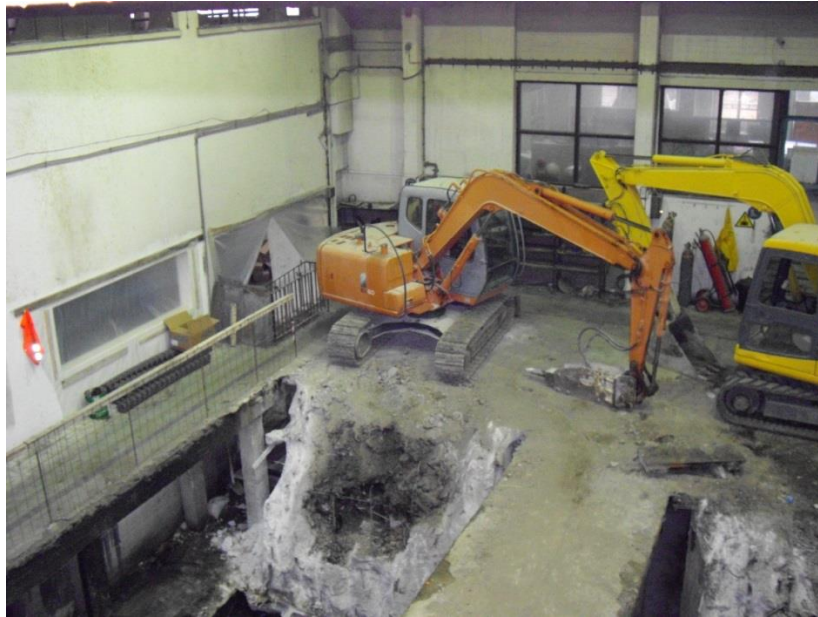
Figure 6-1: Foundation construction for a new Genset
