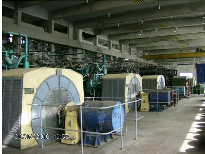
Figure 2-10: Typical engine room arrangement
