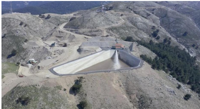
Figure 2-18: NAERA hybrid power plant reservoir
