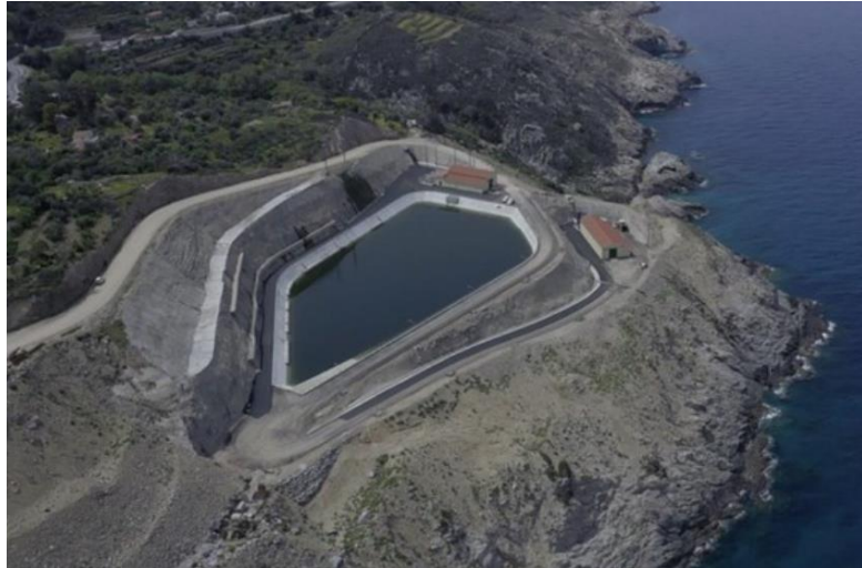
Figure 2-20: NAERA hybrid power plant reservoir
