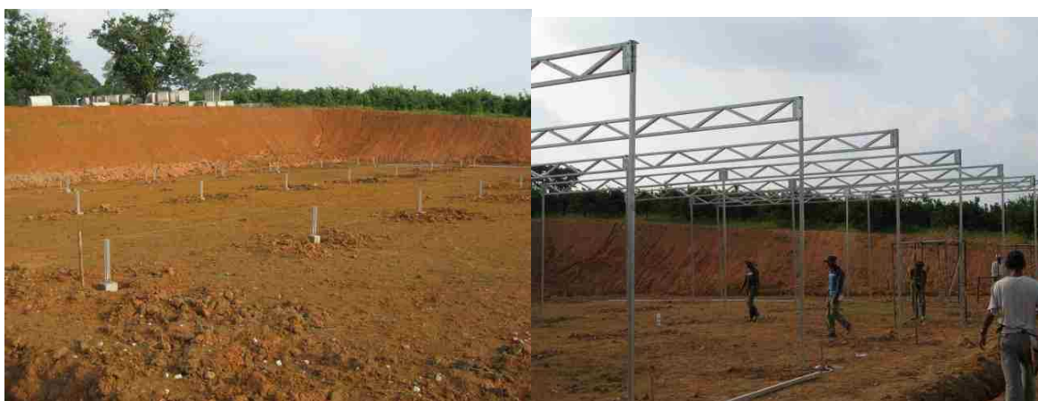
Figure 1. Construction of one of the greenhouses at Serdang.
