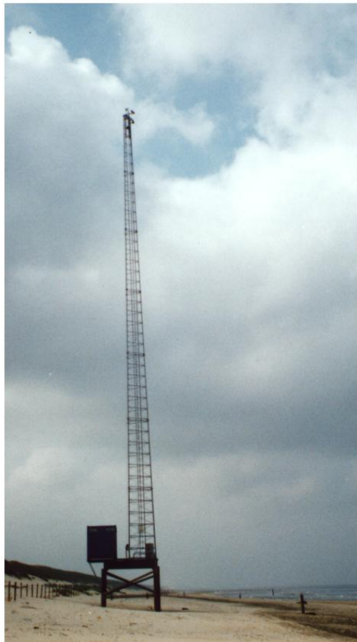
Figure 2 Mast for the Argus station at Egmond-aan-Zee Coast3D beach
