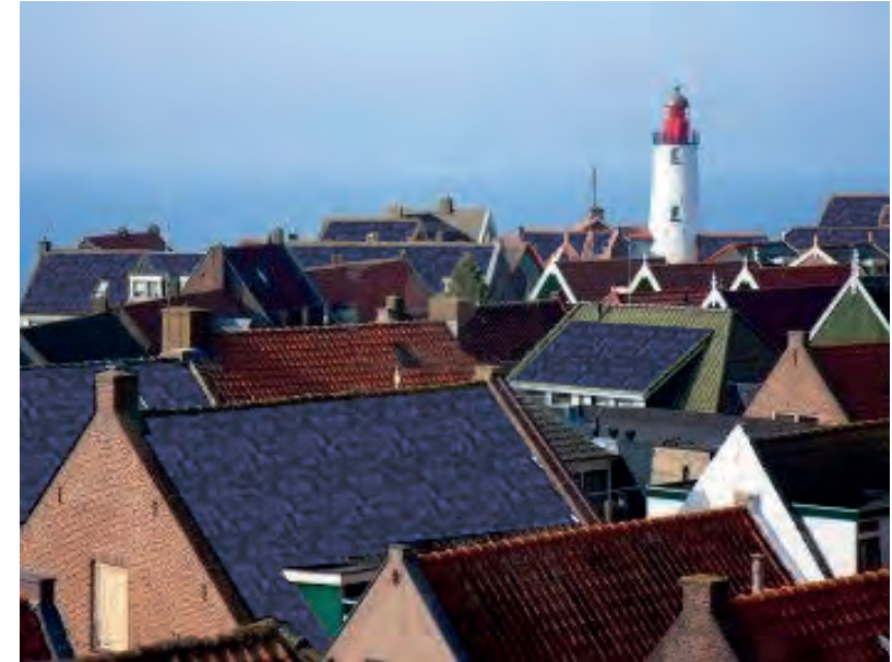
Figure 2.56 Solar panels on existing houses
