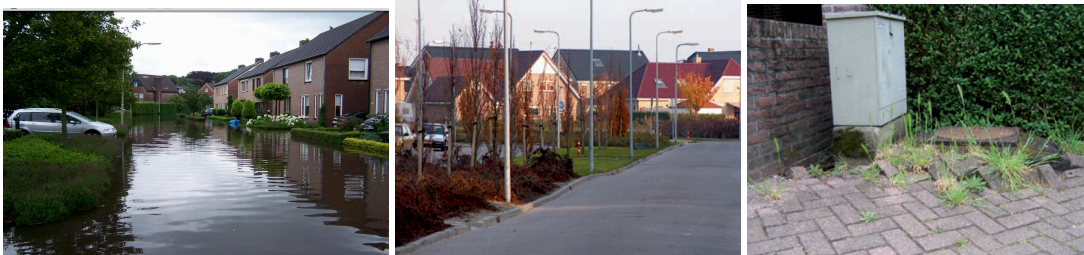
Figure 4. Problems associated with building on peatland, examples from the Netherlands: flooding (left); subsidence of roads (middle), and; subsidence of sewerage mains (right) (Deltaris, 2008)
