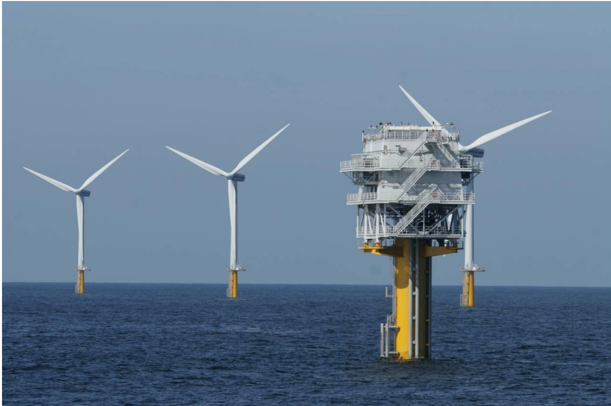
Figure 3. Transformer platform and three of the 60 turbines of PAWP. The PAWP turbines are smaller, but placed closer together than the OWEZ turbines. Note that both the PAWP transformer platform and the OWEZ metmast offer a platform for roosting seabirds, such as cormorants and gulls. Photo: Hans Verdaat, IMARES.
