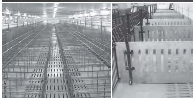
quality concrete flooring and penning
