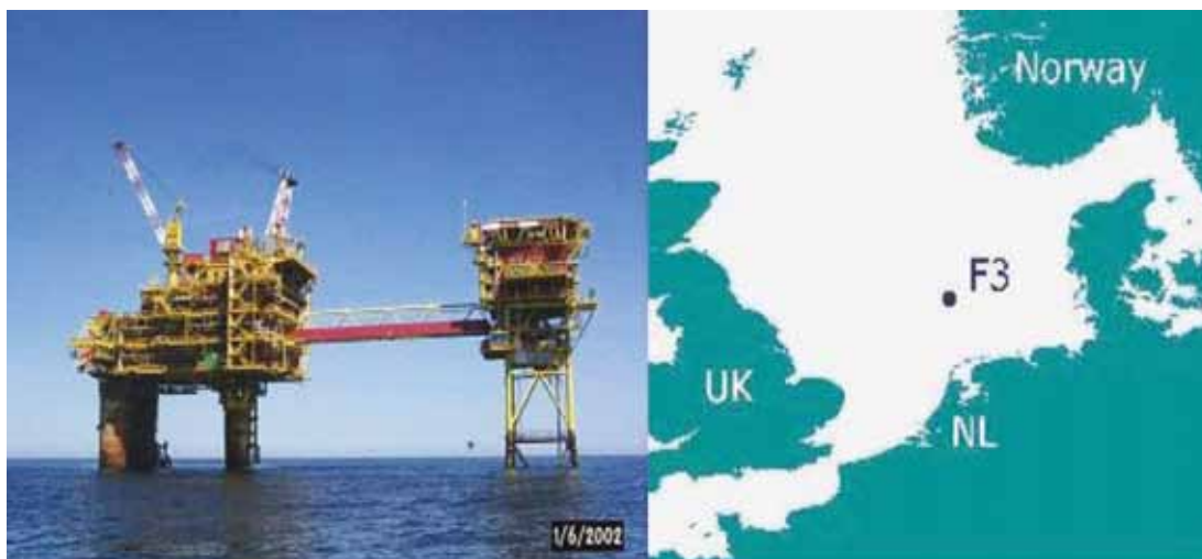
Figure 4.7 The F3 platform (left graph) consisting of the larger actual production platform and the smaller accommodation platform, and its location (right graph) in the central North Sea.
