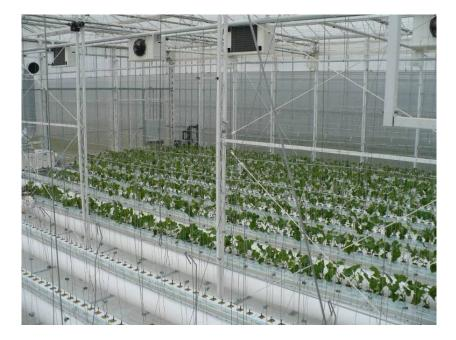
Fig. 3. Heat exchanging units hanging above the crop in the closed greenhouse.
