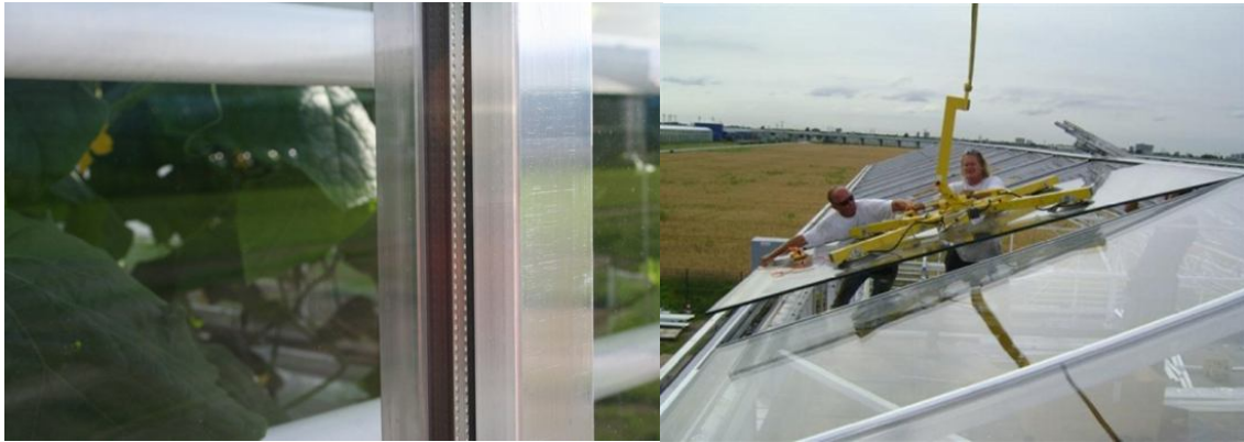
Figure 4.6. Double glazed greenhouse cover with AR coating (3 sides) and low energy coating (1 side)
