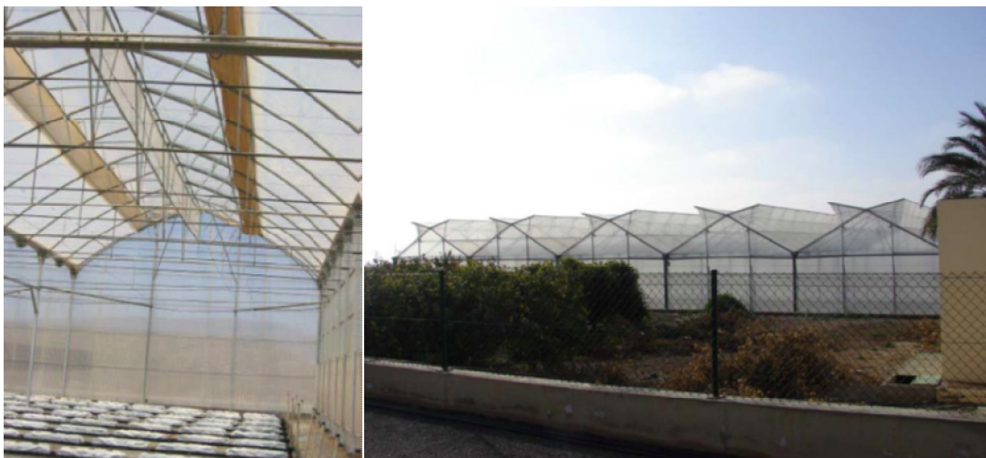
Figure 4.1. New type of multi-tunnel greenhouse with improved ventilation (EEFC, Almería, Spain)
