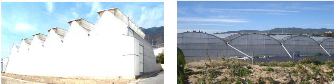
Figure 45. Double sided and single sided roof vents.
