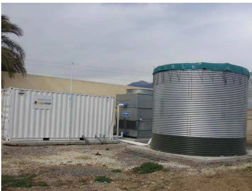
Figure 2.1. Water silo energy store, designed by EEFC to cool and heat a 1000 m 2 greenhouse. The single store is an inexpensive option for the storage of both cold and warm water.
