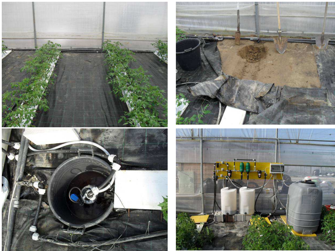
Figure 6.3. The installation of the experimental growing systems set up in the Italy test site greenhouse.
