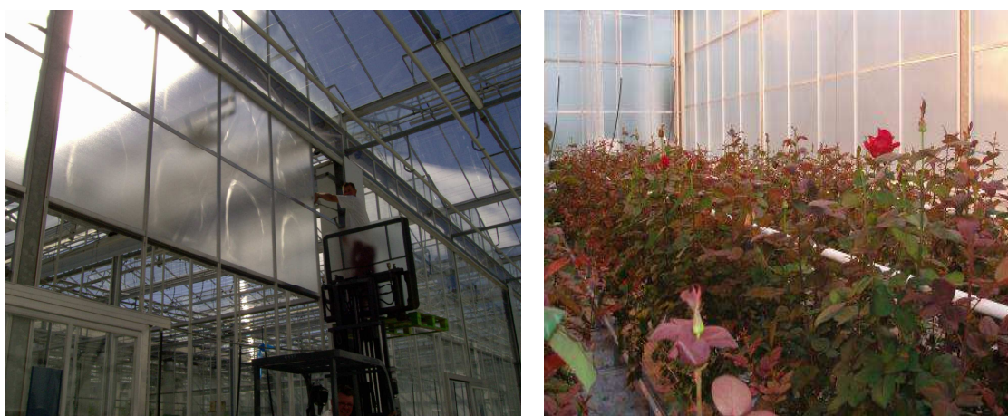
Figure 5.2: the glass has a prismatic structure that makes the light diffuse and reduces the apparent transparency of the glass. Picture left: during the replacement (august 2010), picture right, November 2010, during cultivation.
