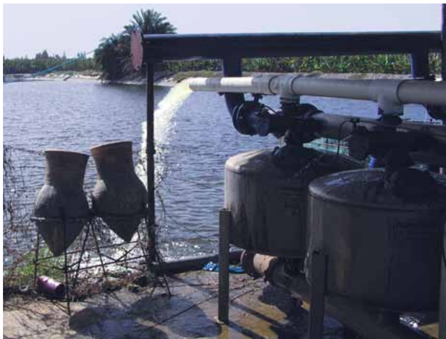
This concrete-lined reservoir for storage of Nile water is stocked with tilapia. The water passes through sand filters (right) before it is pumped into the drip irrigation system.
