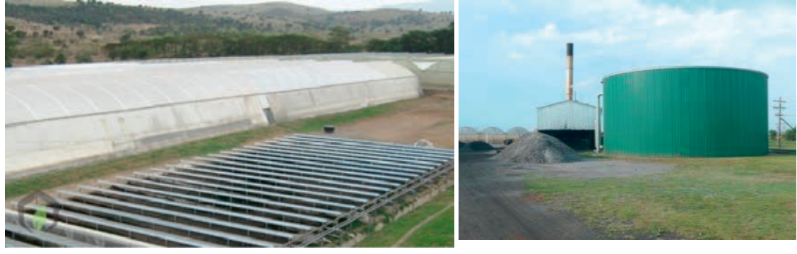
Figure 3.22. a solar collector for greenhouse heating (left; www.certhon.com ) and a heat storage tank (right).
