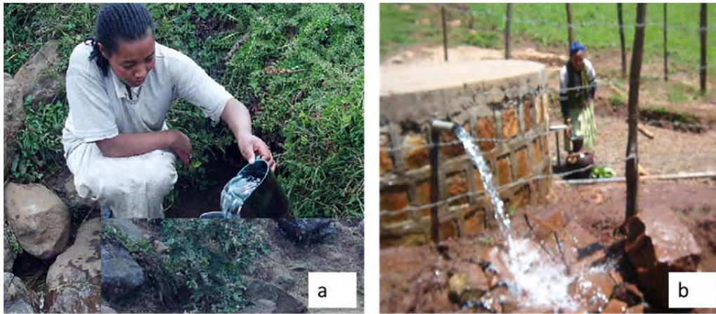
Figure 6.3. A spring before protection (a) and after protection (b) in the Galessa watershed (Lege-abatibo spring), Ethiopia.
