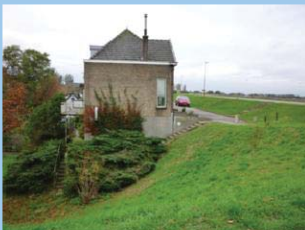
Figure 3.3 As a result of past reinforcements, many historic and characteristic houses are situated against or even on or in the current embankment (photograph: J.M. van Loon-Steensma).
