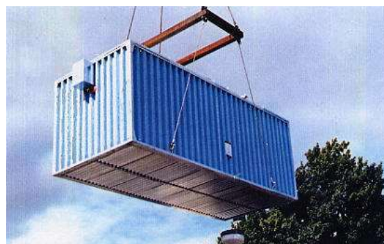
Figure 8 Portable heating and cooling bank
