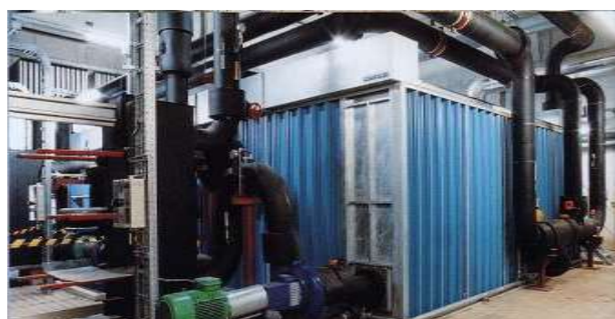
Figure 7 Energy storage, hot water or ice bank, courtesy by FAFCO – www.fafco.ch
