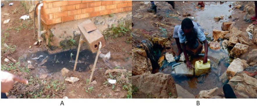
**Figure 9.3:** A) Grey water from a bathroom stagnant beneath a water meter for a piped water supply house connection in Bwaise III and B) Evidence of exposure to contaminated and unprotected drinking water in Bwaise III
