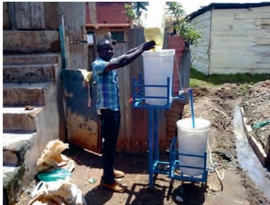
**Figure 9.5:** A crushed lava rock filter for grey water treatment by a household in Bwaise III
