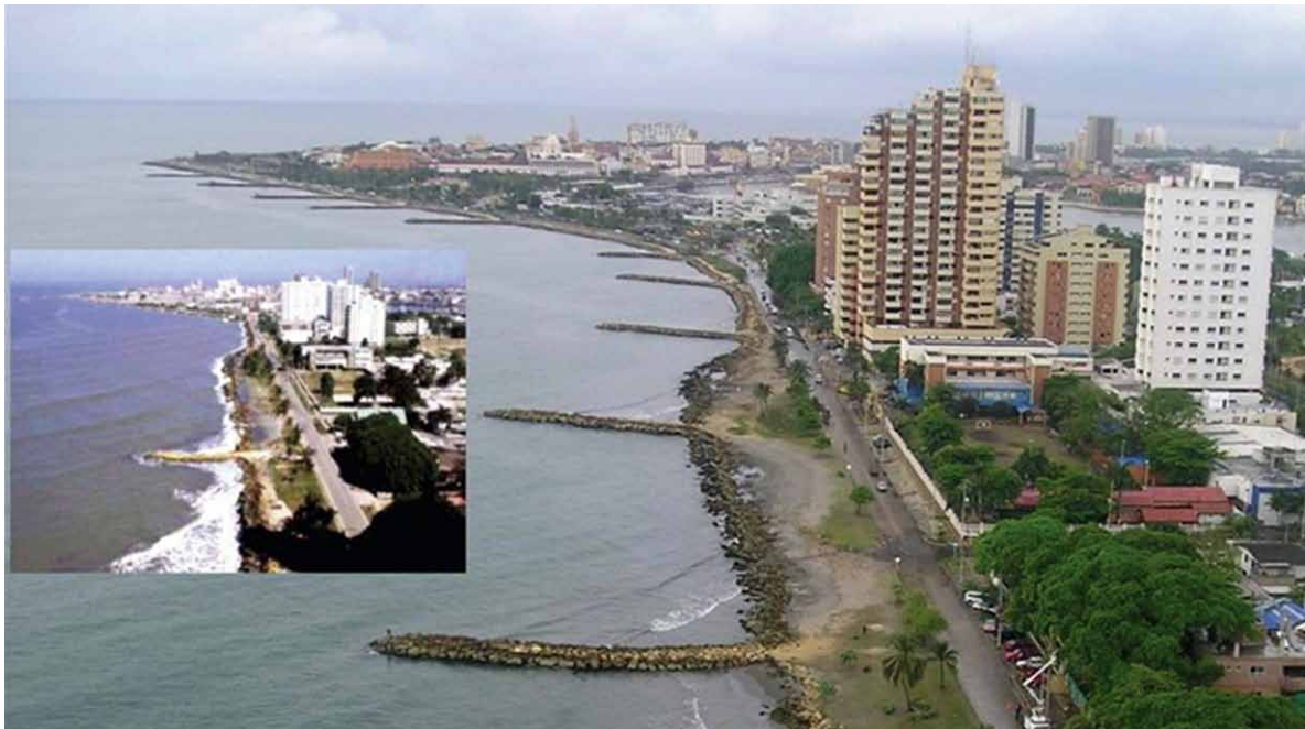
Figure 2 Coastal erosion at Cartagena. 2
