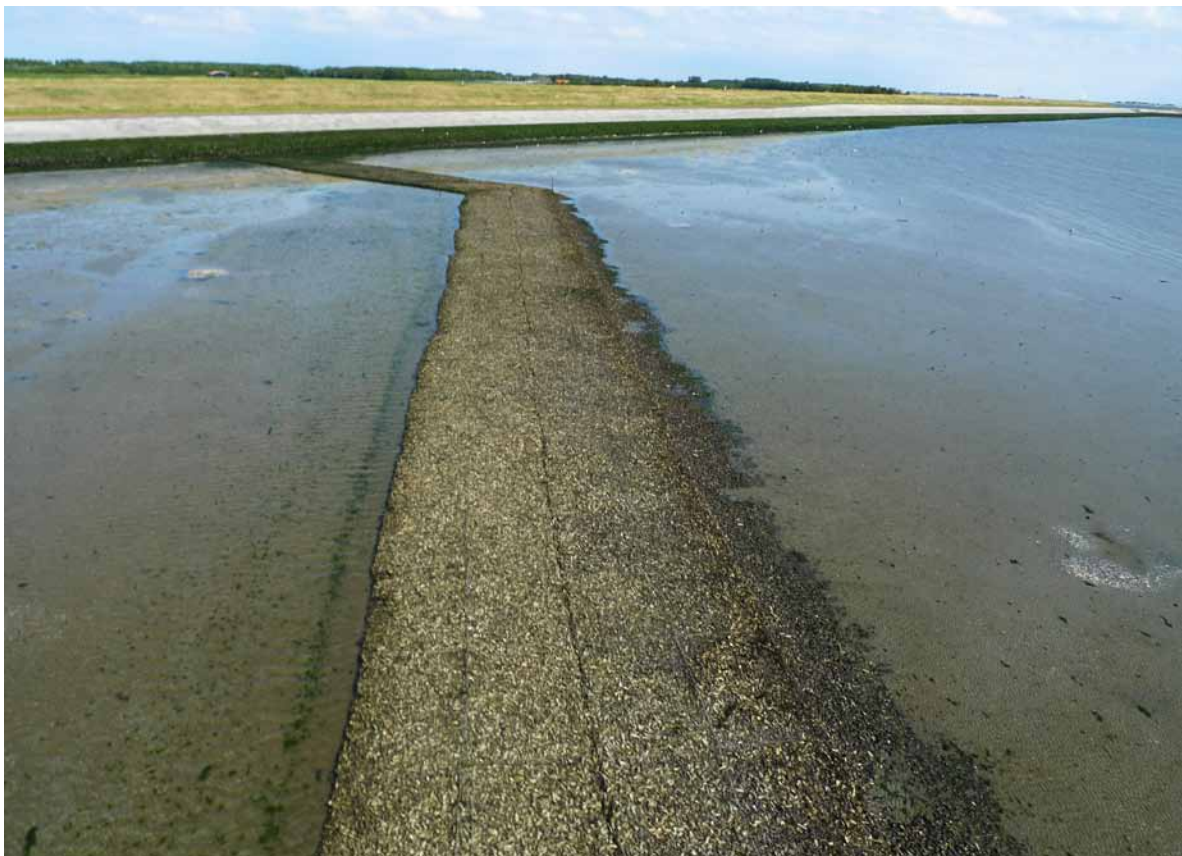
Figure 4 Oyster reef functioning as a breakwater and sediment stabilizer.
