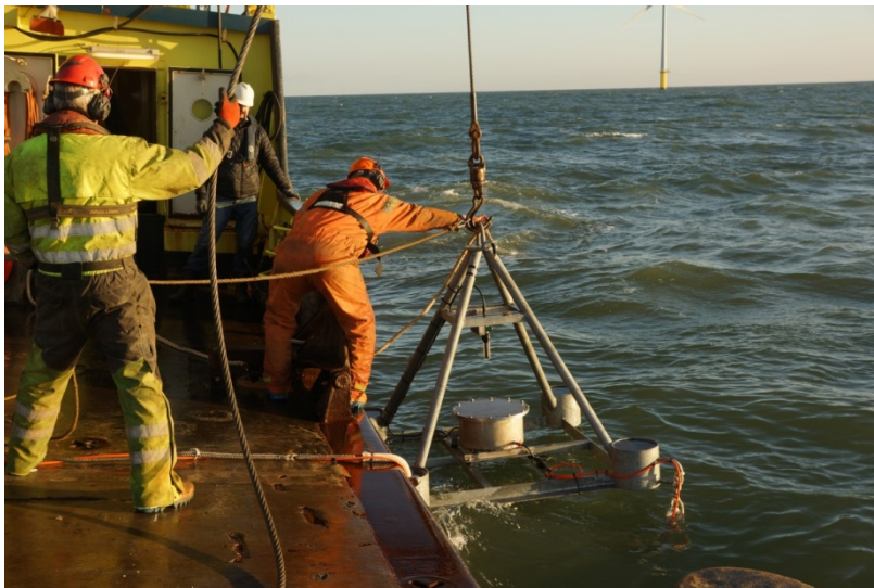
Figure 14 Deck operations on board MS “Terschelling” shortly before the deployment of the equipment in the OWEZ wind farm 100m east of WTG27.
