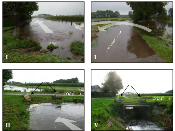
Figure 3.11: The role of culverts during the 27 August 2010 flash flood. The roman numbers indicate the post-event field surveys (Table 3.1). Upper panels: Situation directly after the flood. Upwelling water reveals the exit of the submerged culvert. The resulting backwater feedback allows water to bypass the obstacle on the right by flowing over the road and the adjacent field back into the brook (arrows). Lower left panel: upstream entry of the culvert. Logs (black arrows) deposited by flood and flow marks in grass (upper left panel) indicate that water flowed over the culvert at flood peak. Lower right panel: situation two weeks after flood with flood marks indicated. The photos in the top panels of Fig. 3.7 are taken from the same location as the photos in this figure, but in upstream rather than downstream direction.
