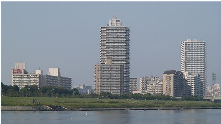
Figure 6: Example of a super dyke with high rise buildings in Japan. ( www.kennislink.nl )
