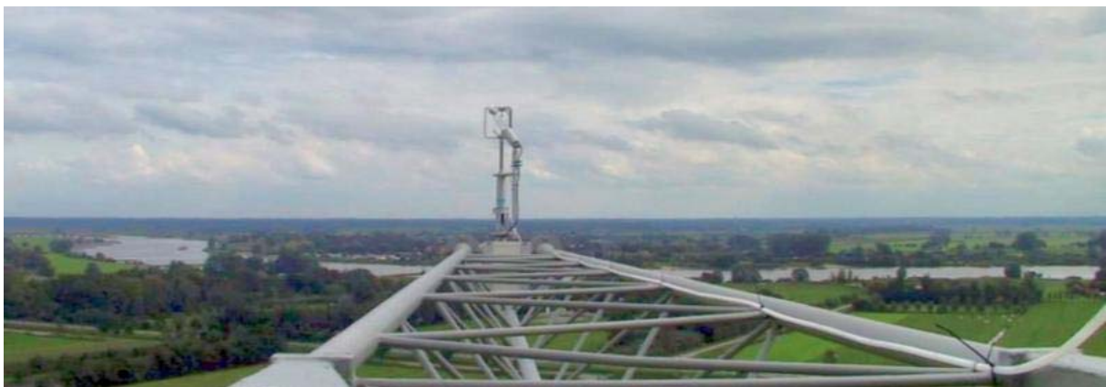
One of the tower measurement booms at the Cabauw .
