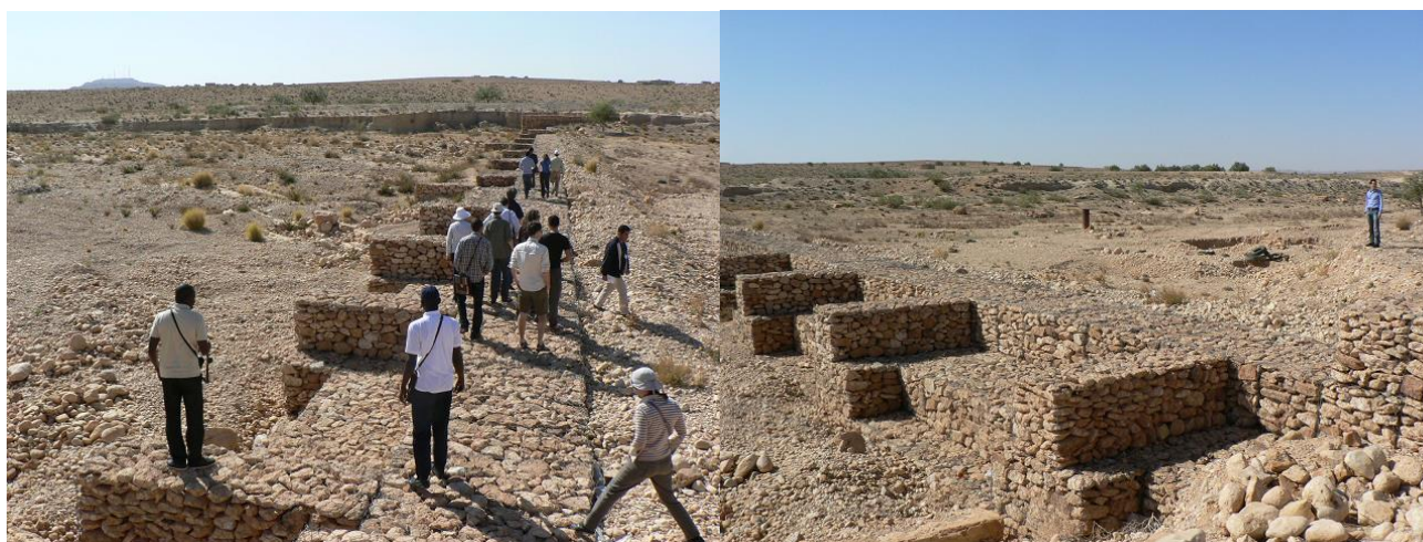
Figure 1.1: Two pictures of the same check dam in a dry river bed in the Oum Zessar watershed. Since flow is from right to left, the retention basin is directly to the right of the dam. Pictures taken by author.
